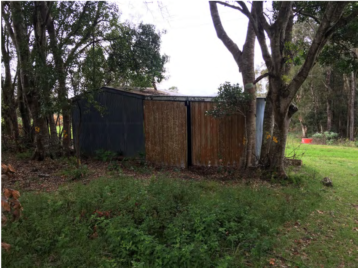
Photograph 5: View south of rear of 1986 tractor shed. The cladding is metallic. The right hand side appears to be an extension beyond the 1986 building application. The floor is exposed soil.
