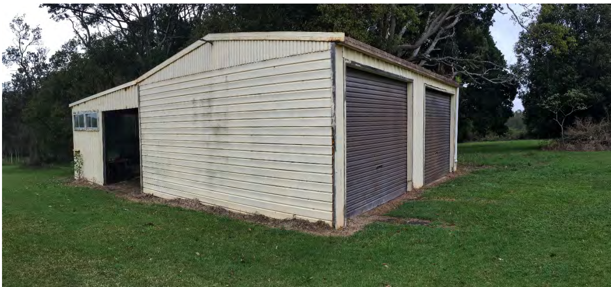
Photograph 3: View south-west of 1982 shed plus 1986 extension at the rear. The cladding is metallic. The floor of the rear part of the shed comprised exposed soil. The closed section of the shed was not accessed but is likely covered with 100mm concrete based on the 1982 building application.
