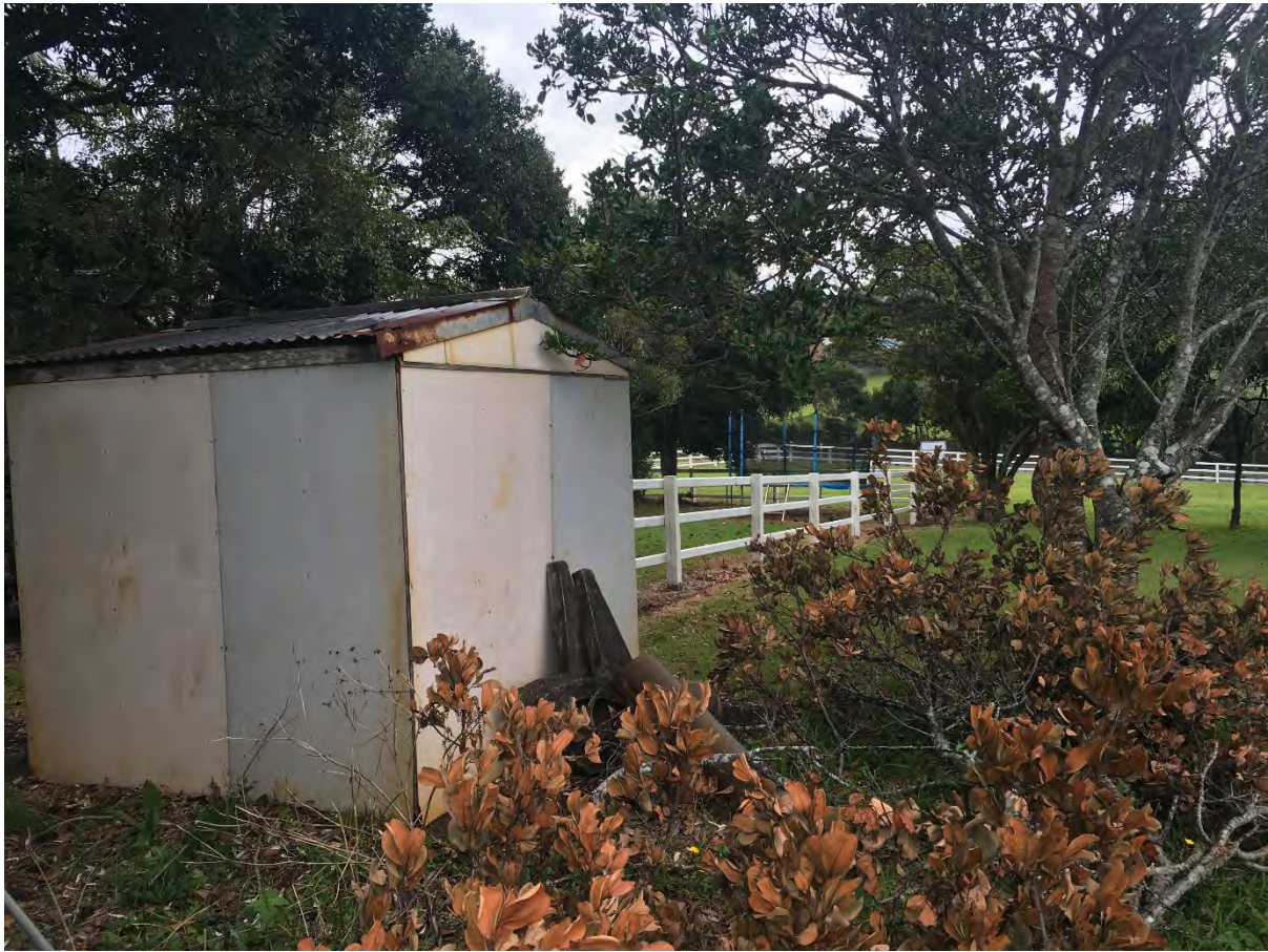
Photograph 11: View north-west of small shed located to the east of the dwelling. The roof is metallic however the wall cladding is likely fibre cement sheeting, although positive identification of whether the cladding contained asbestos fibres was not possible. Note the concrete pipe and collars stacked against the shed.
